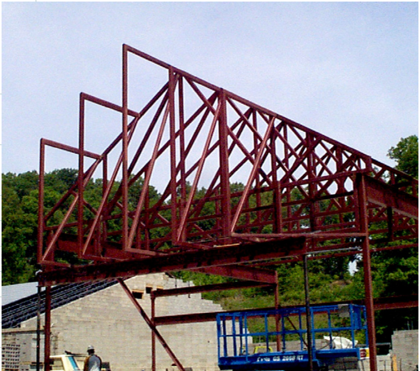
Classroom wing under construction
